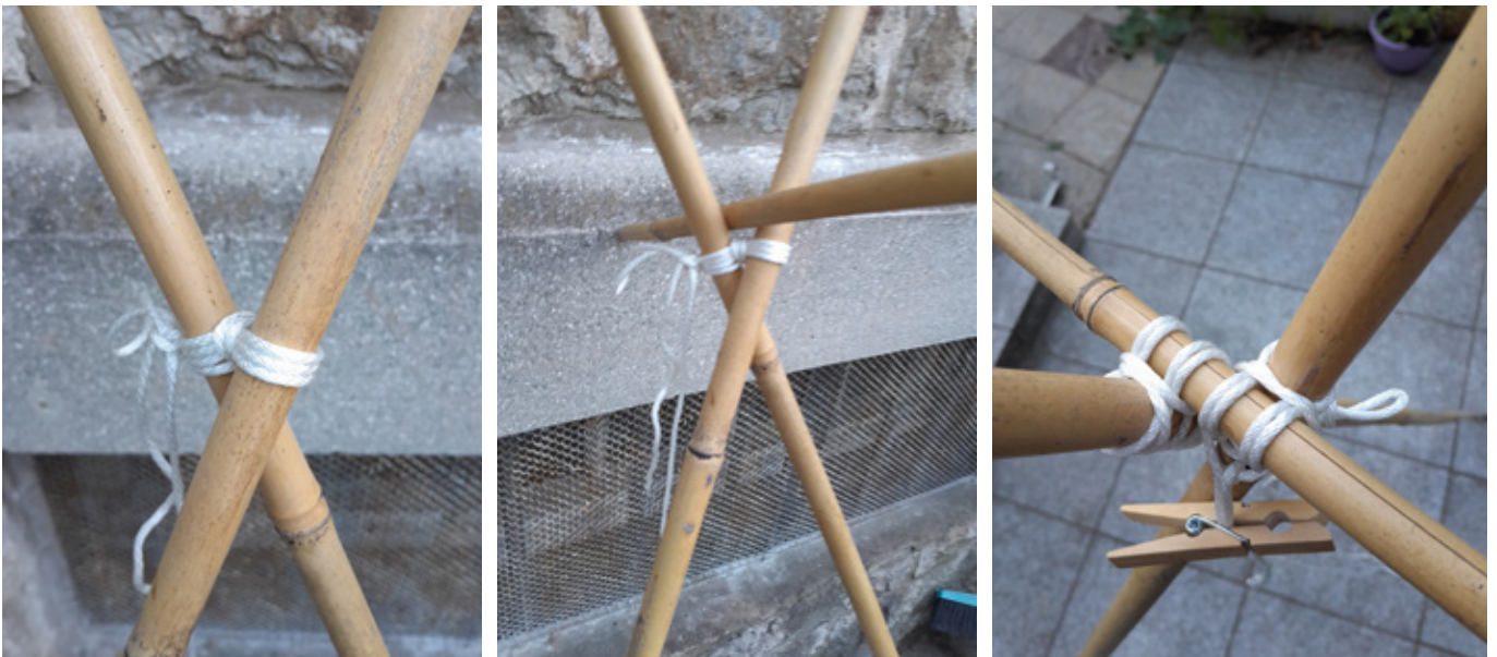
Positioning and knotting the top horizontal pole
